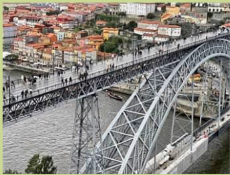
Upper and Lower levels of the bridge
